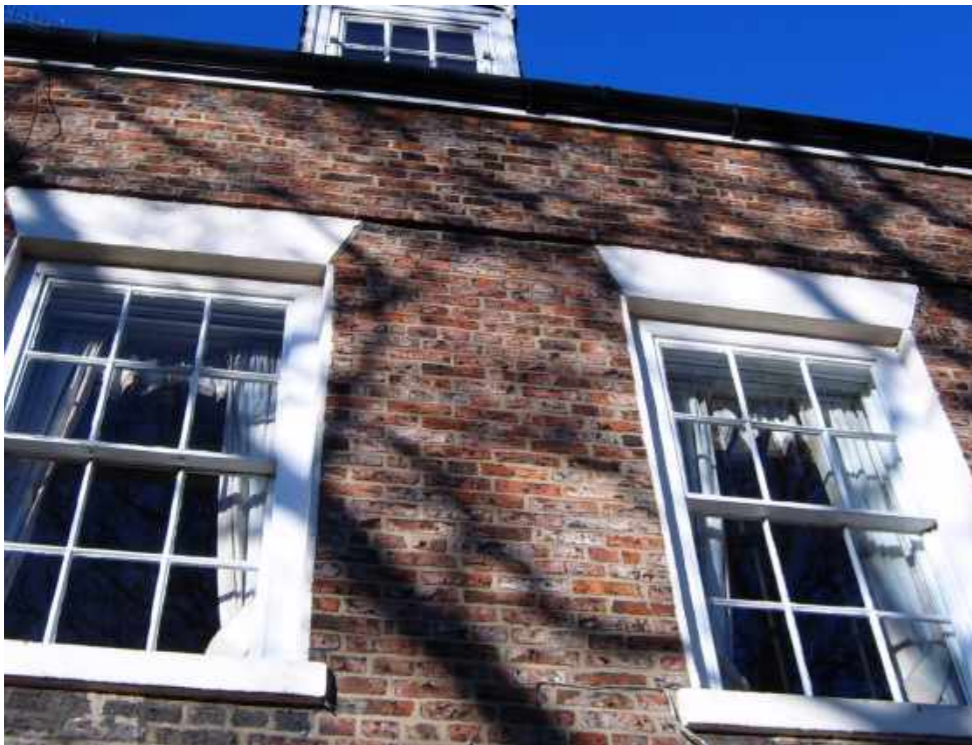
EXAMPLES OF THE EXISTING TIMBER SASH WINDOWS
