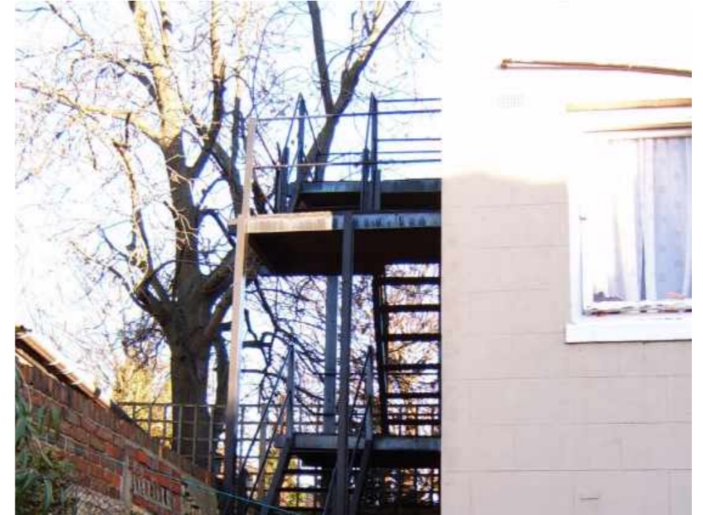
EXISTING STEEL FRAME FIRE ESCAPE LOCATED AT THE REAR OF THE EARLY GEORGIAN TERRACED UNITS
